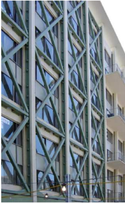
FIG 14.2.1-A Infill shear trusses -University of California dormitory, Berkeley
