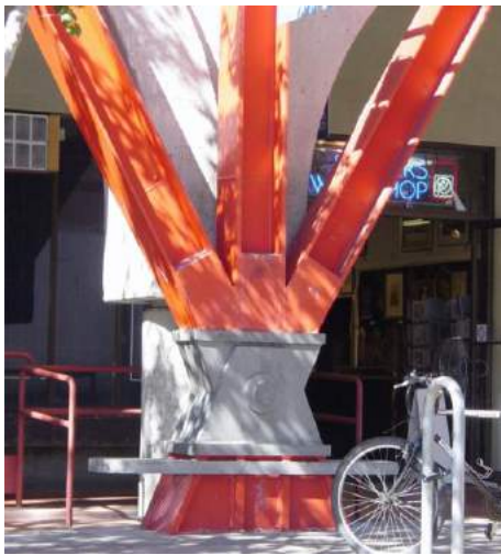
FIG 14.2.1-B External bracing of an existing reinforced concrete parking garage (Berkeley)
