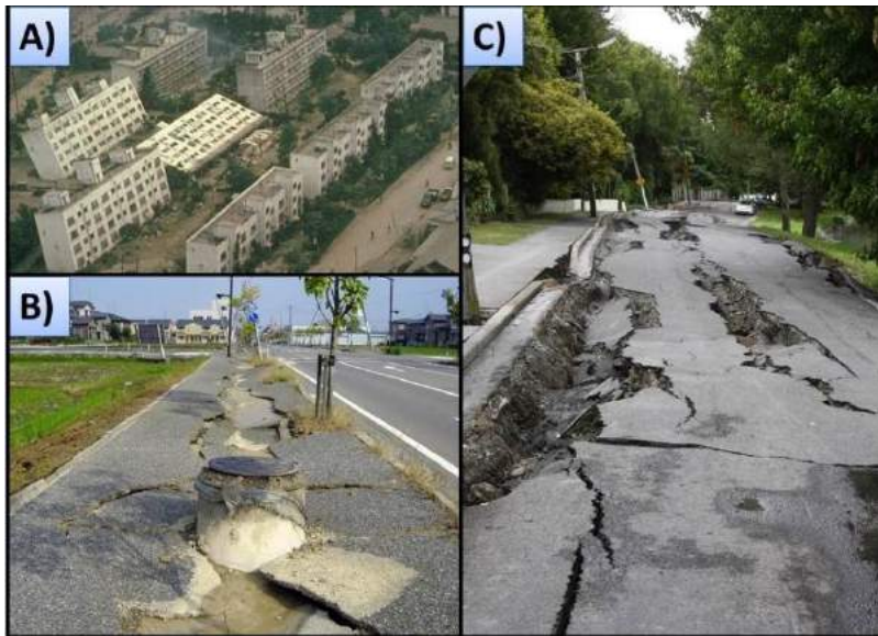
Fig 5.1.2.B due to soil liquefaction
